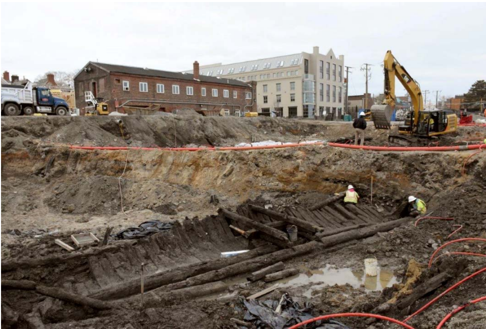
RTS Ship #2, unexcavated overview. Wharf cribbing fragment visible approximately amidships. Courtesy of Alexandria Archaeology.
