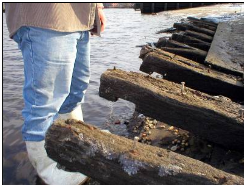
Frames showing limber holes.
