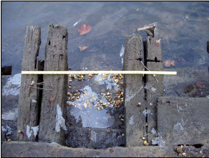
Detail of frames showing spacing and fastener pattern.
