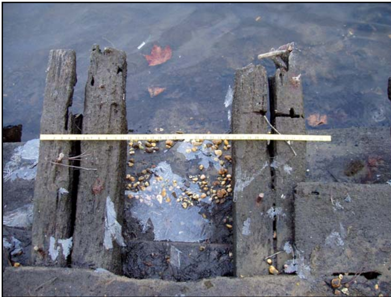
Figure 6. Site 18WC185, frames, ceilings, and outer hull planking.
