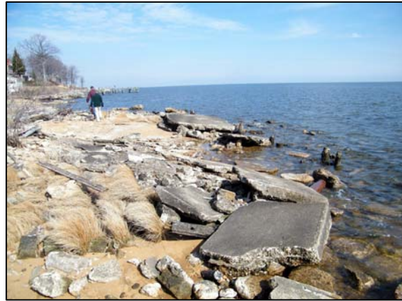
Figure 6-24. Concrete Slab and Piers of the Pinehurst Pavilion Today.
