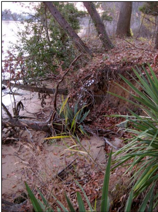
Figure 5-65. Shell Eroding from Bank at 18AN1005.
