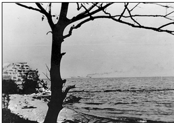
Base of Bodkin Light tower (date unknown).
