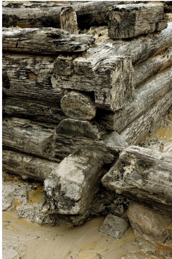
Detail of a bulkhead wharf at the Robinson Terminal South Site. Unless noted, all images courtesy of Alexandria Archaeology.
