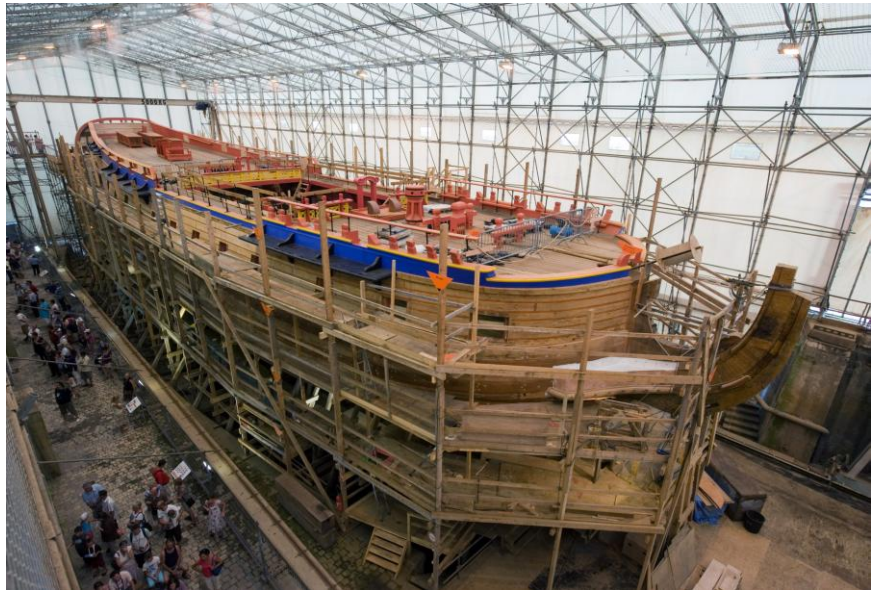
Tours were conducted during the construction at Rochefort. Photo: CMT-S.Sciot.
