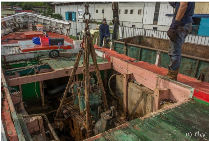
Crane operator removing the diesel engine. Photo by M. van Veldhoven.
