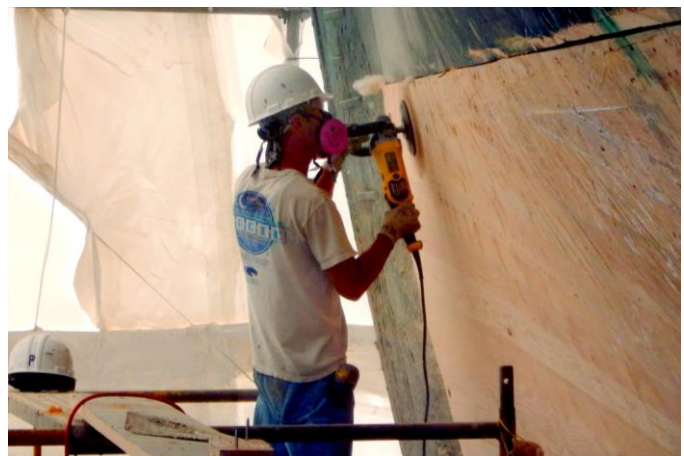
R. Howard sands the bow planking. After sanding, oakum will be installed in the joint above, and the planks will be primed and painted, all to keep the ship watertight for the next 20 years. Photo by J. Smailes.
