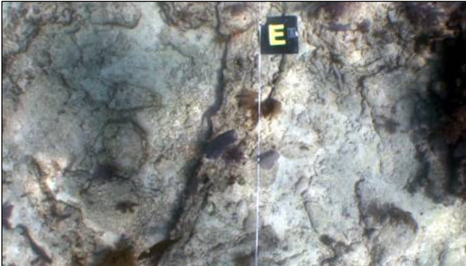
Railing, to the left of the video lane centerline.
