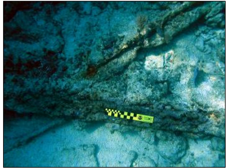
Metal framing: scale is in 1- and 2-centimeter increments. Photo by J. Smailes.
