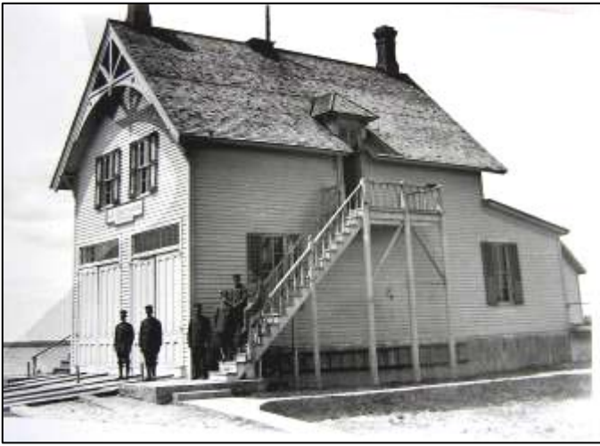
Boathouse and Keepers House at MILSS. Photo courtesy of the Great Lakes Lighthouse Festival Museum.
