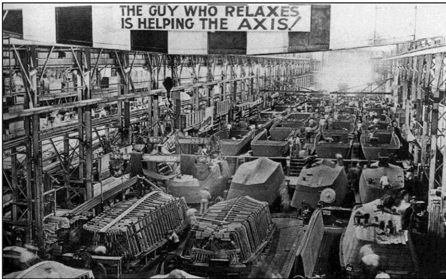
Moving assembly line with LCVPs in foreground upside-down: note the V-shaped bow and reversed curve of the stern.
