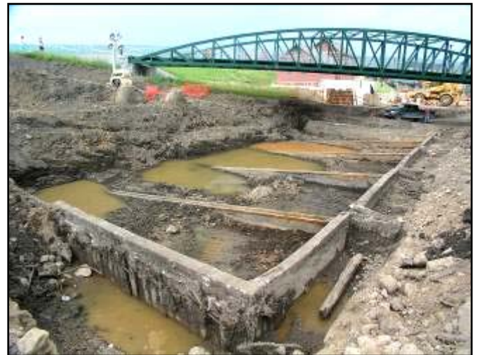
Overview of the Canal Towage Company Marine Railway, facing north. Photo by J.Balicki
