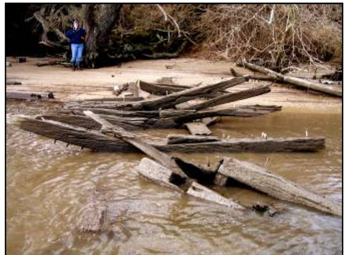
Schooner or bugeye at Patrick's Landing. Frames are notched to fit over the keel. Photo by E. Ragan.
