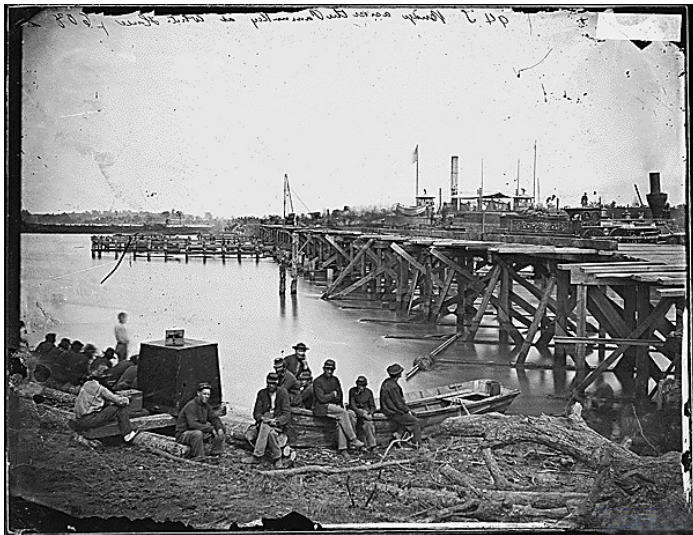
Bridge over the Pamunkey River at White House Landing under repair ca. 1862, with locomotive in right background.
