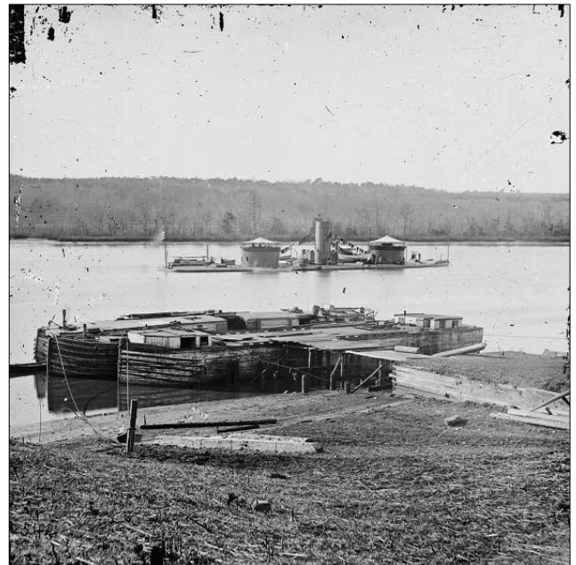
Barges moored parallel to the shoreline to create a temporary wharf, with a double-turreted ironclad in the background.
